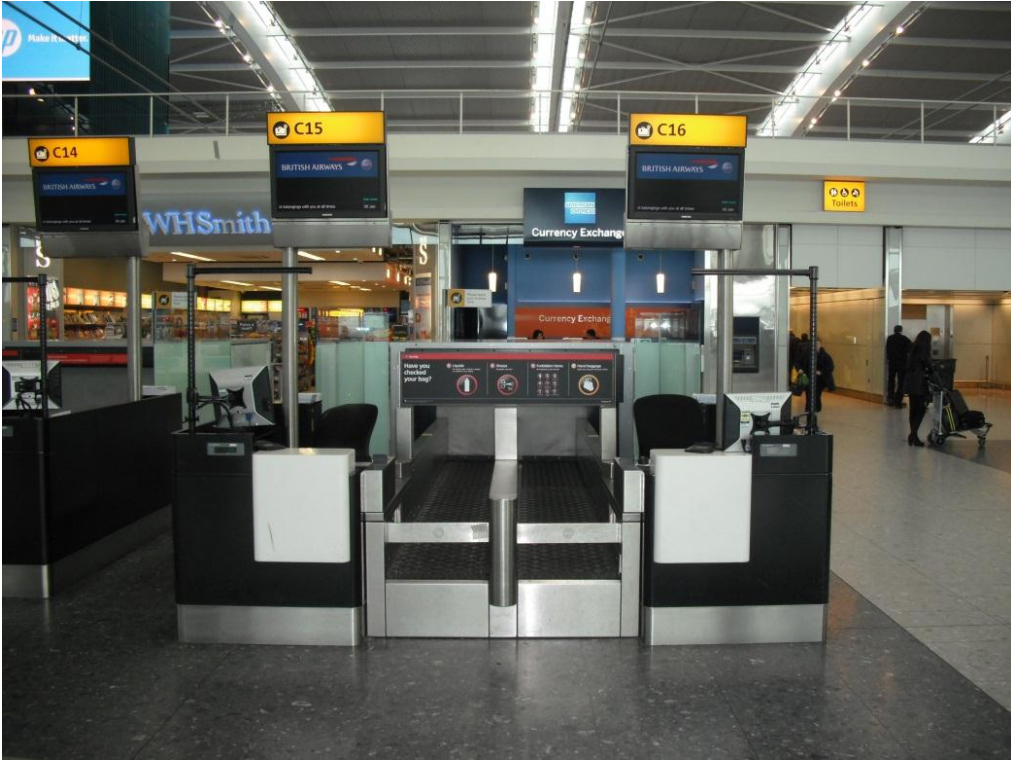
Existing Manned Bag Drop Desks. One pair to be removed (location tbc) and replaced with a pair of self-service bag drop units
