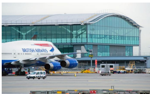
Terminal 5C External view
