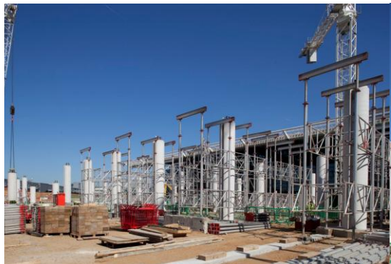
Multi Storey Car Park: Ramp bridges
