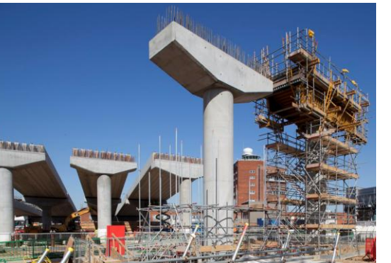
Columns and formwork
