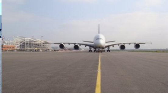
Last section of southern A380 taxiway complete
