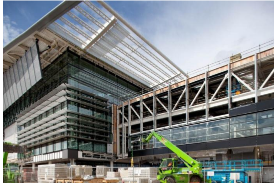
South east corner
