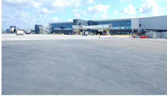
Stands 231, 232 and 233 operational
