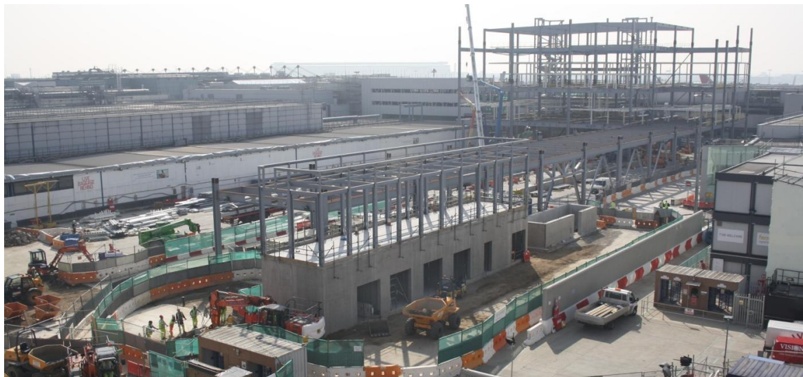
Post T5 Transfers Baggage System
