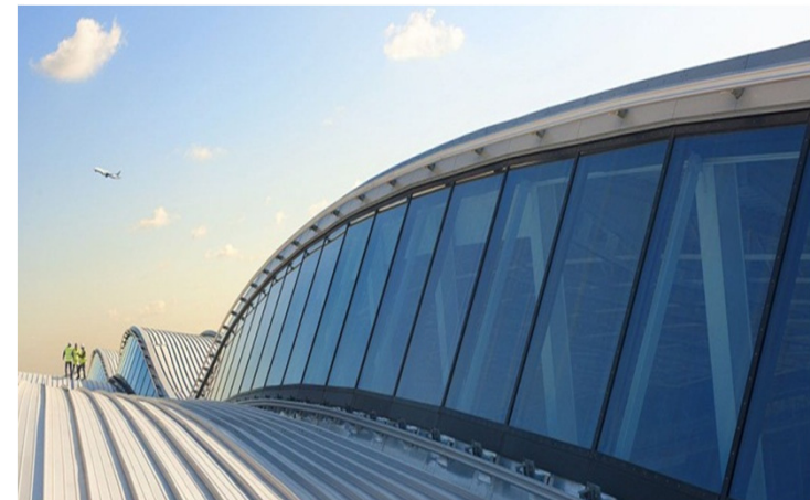
Roof of main Terminal 2 building
