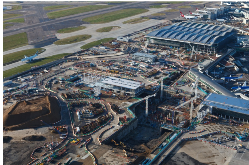
Terminal 2 site – January 2012
