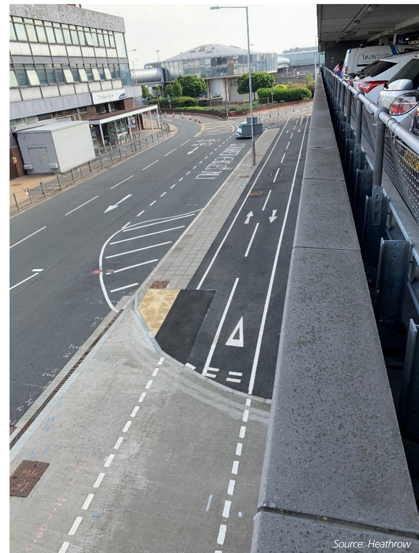
Figure 6: Existing bi-directional cycle track in the CTA
